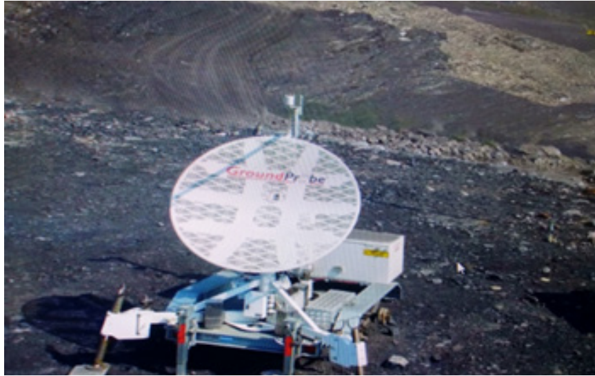
Figure 5 SSR installed in Kusmunda Mines, SECL and India 23 .
