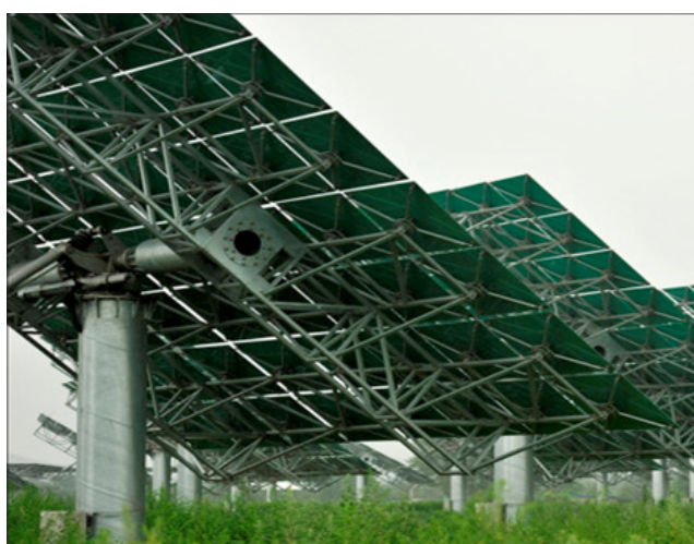
Figure 9. Heliostats in the Dahan concentrating solar power plant in Beijing, China.
