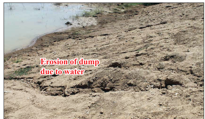
Fig.6: Showing erosion in mine OB dump (as on 15/10/2018)
