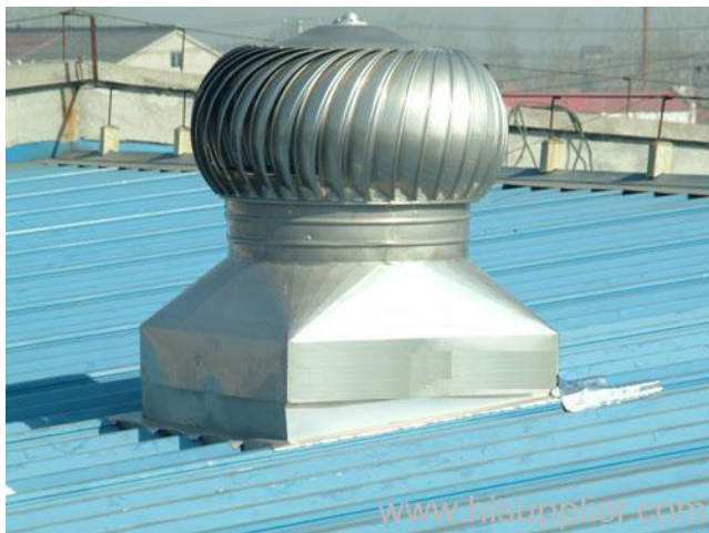
Figure 8. Wind-driven ventilators.
